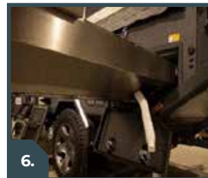
6. WASTE PIPE EXTENDED
